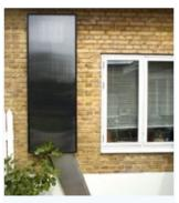
A tube can be used, if the basement is placed too far in the ground for a direct injection.
