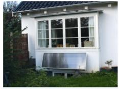
Mounted with an angle the injected air will have a higher temperature during the summer - and thus a more effective dehumidification.
