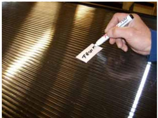
6. Be aware that the surface on the outside and the inside of the cover layer has a slightly difference. It is hard to see therefore make a small note on the outside of the cover layer before removing.
